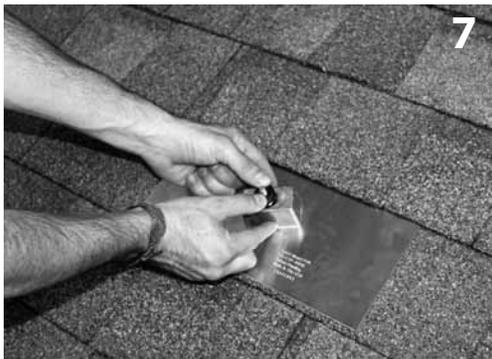
7 Insert EPDM Rubber Washer over Hanger Bolt into Block.
