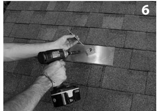
6 Slide Mount back into position. Prepare Hanger Bolt with 1 Hex Nut and 1 Sealing Washer, insert through Block into hole and drive Hanger Bolt into rafter, tightening to a solid snug fit.
