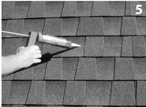
5 Clean off any saw dust, and fill hole with Sealant.
