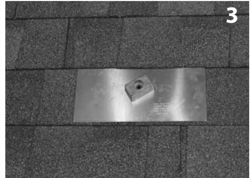
3 Slide Mount into desired position. Remove any nails that conflict with getting Mount flush with front edge of shingle course. Mark center for drilling.
