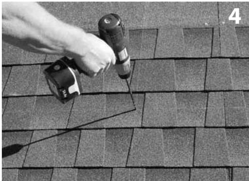
4 Using drill with 7/32" long bit, drill pilot hole into roof and rafter, taking care to drill square to the roof. Do not use Mount as a drill guide.
