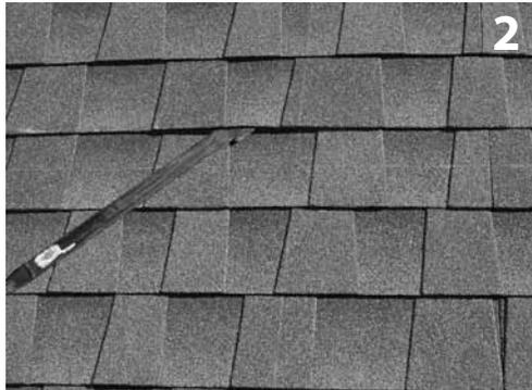
2 Lift Composition roof shingle with Roofing Bar, just above placement of Quick Mount.
