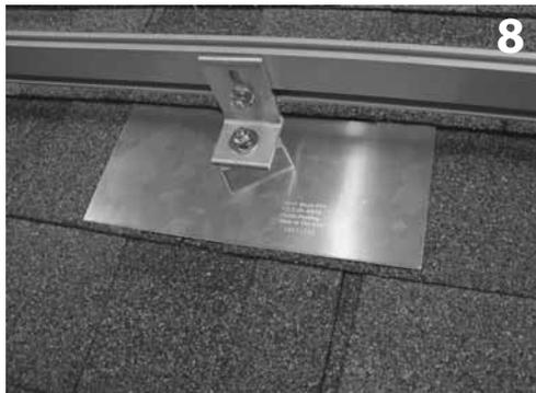
8 Using the Rack Kit Hardware, secure the rack of your choice (see 9\*). Tighten to 13 foot Pounds.
